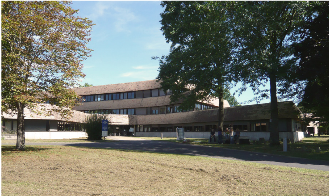
Entrée principale avant travaux Main entrance prior to works
