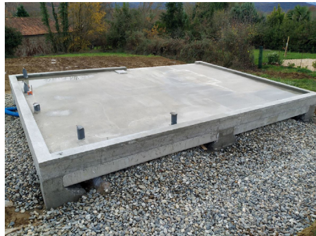
4.2 Fondations, dalle béton hourdis, élévation ossature bois © cosma architecture
