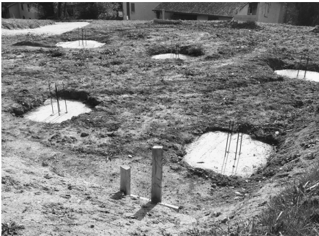
4.2 Fondations, dalle béton hourdis, élévation ossature bois © cosma architecture
